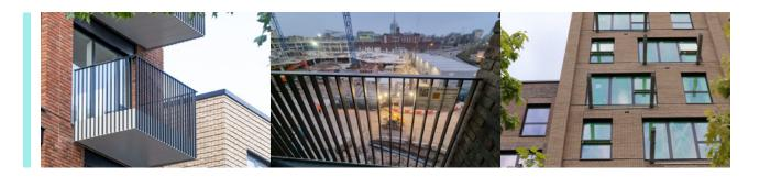
able to manufacture offsite brick columns for corner balconies, inset balconies, and balconies with brick slip fascias. These components were mechanically fixed offsite with brick slips, enabling them to blend effortlessly with the rest of the brick facade, mirroring the industrial aesthetic of the former factory.
