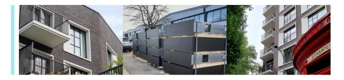
To achieve a contrasting appearance, Sapphire leveraged its expertise in aluminium balustrade railing designs, complementing the GRC balcony fascias manufactured specifically for this project. These fascias were provided with cast-in fixings, allowing for seamless integration with Sapphire's balcony systems. This approach enabled a unified look that contributed significantly to the building's overall aesthetic.
